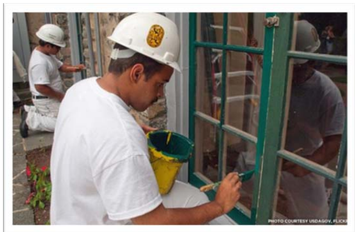
Workers Restoring Historic Windows
