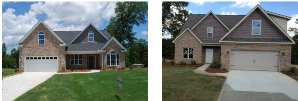
Figure 12: Example of a typical Jones County suburban residential subdivision
