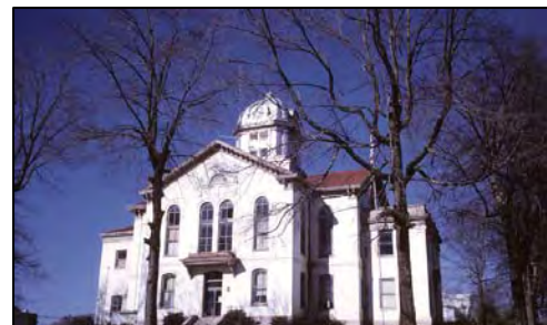
Jefferson is working together with Jackson County on a plan for the historic Jackson County Courthouse
