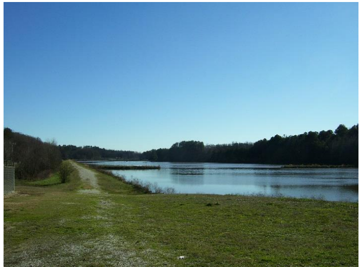
Curry Creek Reservoir
