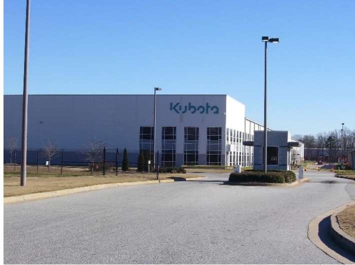
Kubota Building Addition
