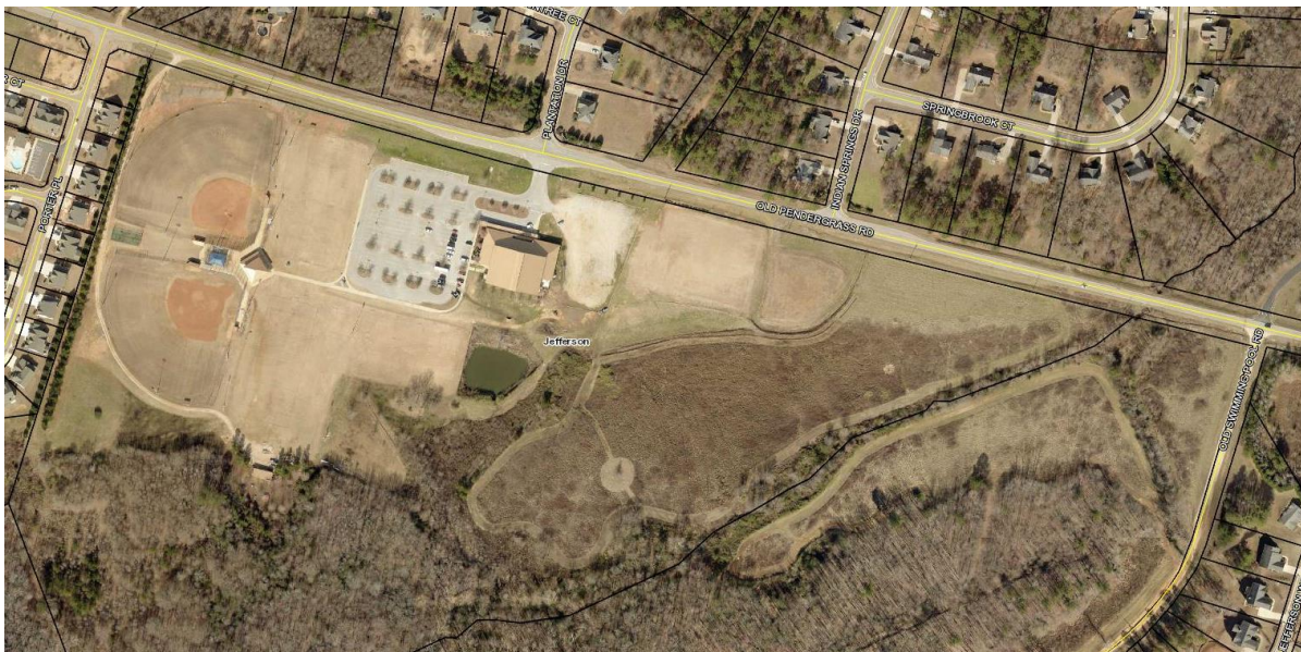
Jim Joiner Recreation Complex (Existing Conditions)
