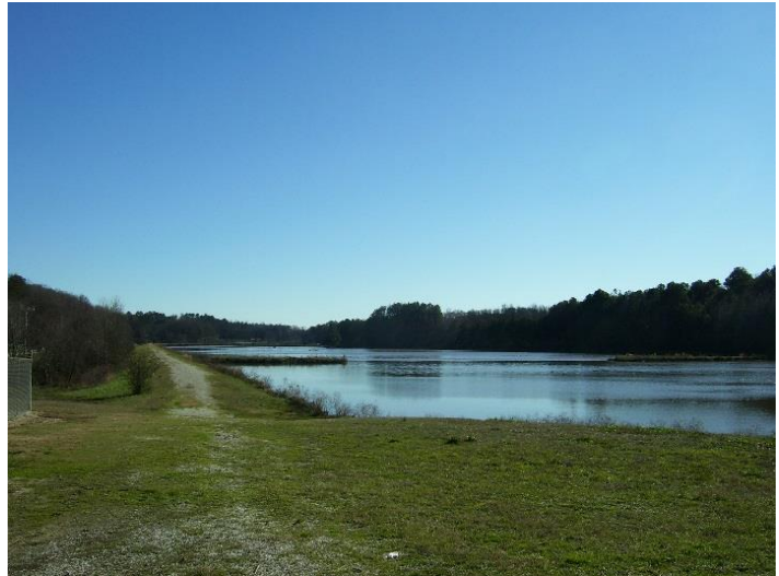
Curry Creek Reservoir
