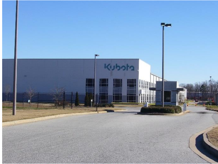
Kubota Building Addition
