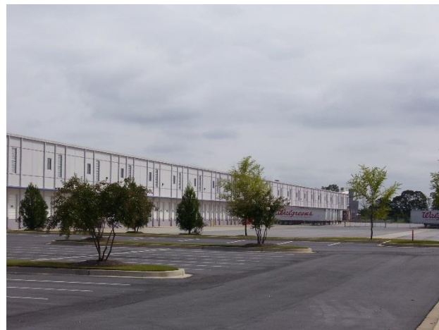
Distribution Center in Jackson County
