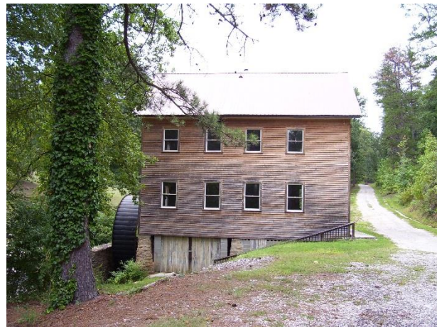
Sells Mill, restored by Jackson County
