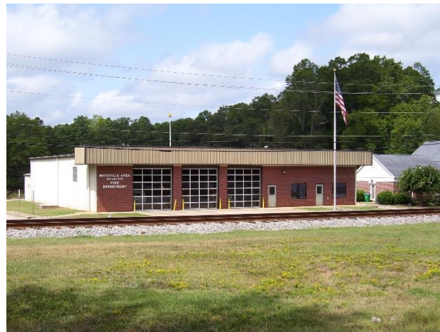
Maysville Area Fire Station
