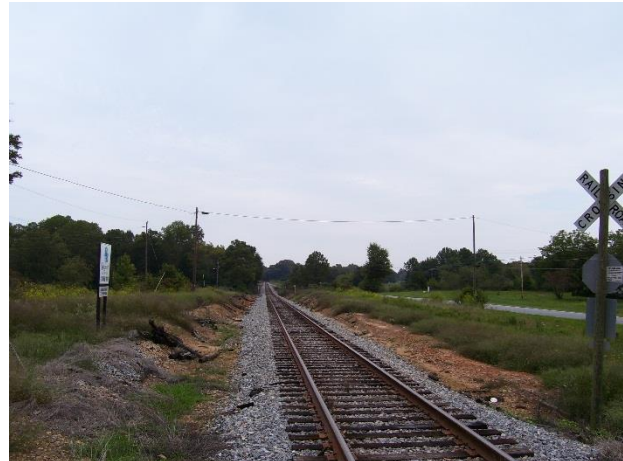
Railroad Between Commerce and Maysville
