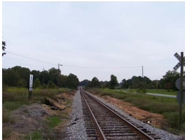
Railroad Between Commerce and Maysville
