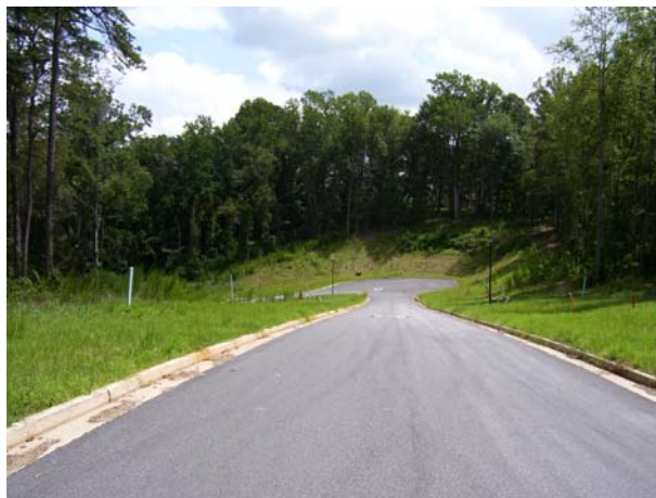
This subdivision, located east of SR 124 just north of SR 11, was constructed on steep slopes.
