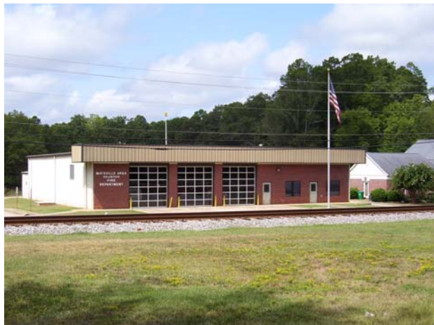
Maysville Area Fire Station
