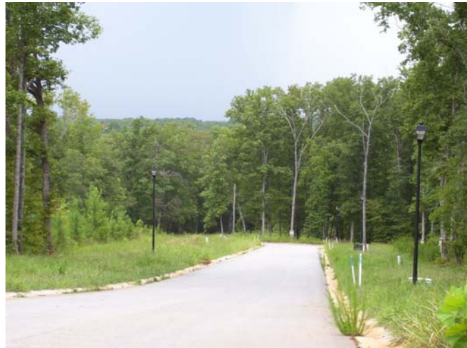
This vacant subdivision street in the River Bend Subdivision is representative of literally dozens of subdivisions that lie mostly or totally vacant; victims of excess subdivision, a flat housing market economy, and subject to vandalism and theft.
