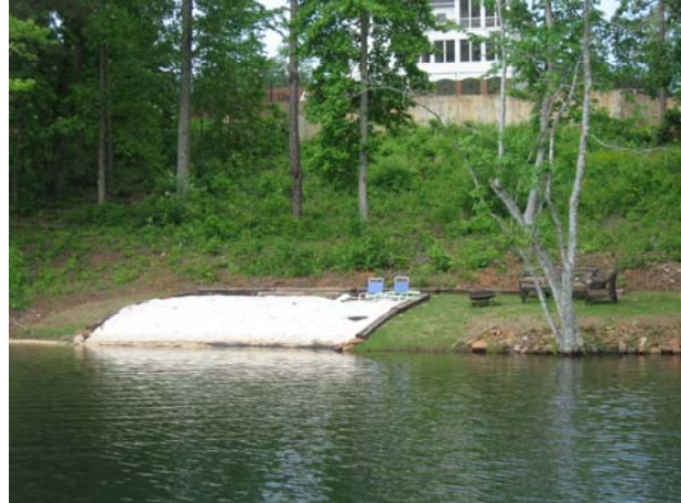
Unauthorized beach constructed within required 150 foot wide buffer for Bear Creek Reservoir
