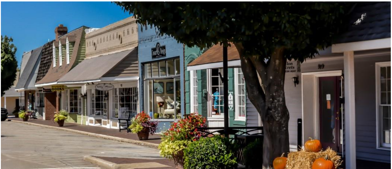
Figure 24 – Historic storefronts in the Perry town center.
