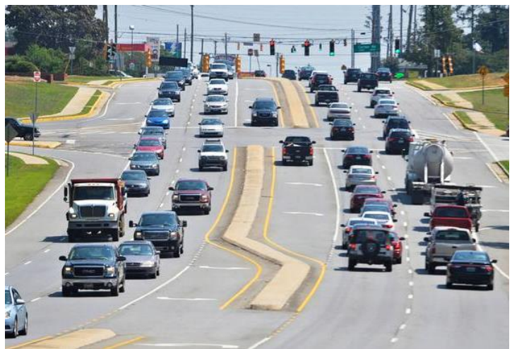
Figure 6 – The eastern stretches of Russell Parkway illustrate several common transportation challenges. Occasional heavy traffic, a lack of pedestrian accessibility, and few aesthetic improvements.
