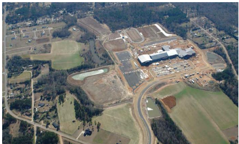
Figure 16 – Aerial photo of construction of Veterans High School in 2009. Note the difference in scale between new school and nearby community in Kathleen.
