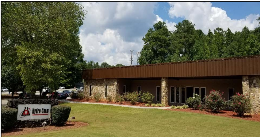
Hydro-Chem, Hickory Springs Industrial Park
