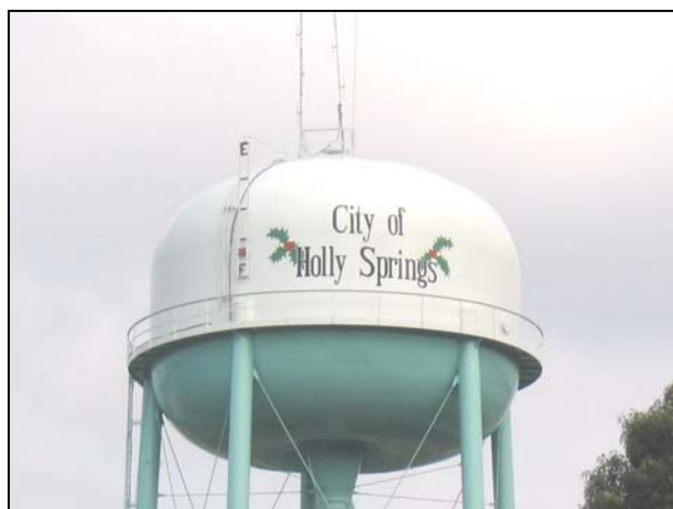
Water Tower, Holly Springs
