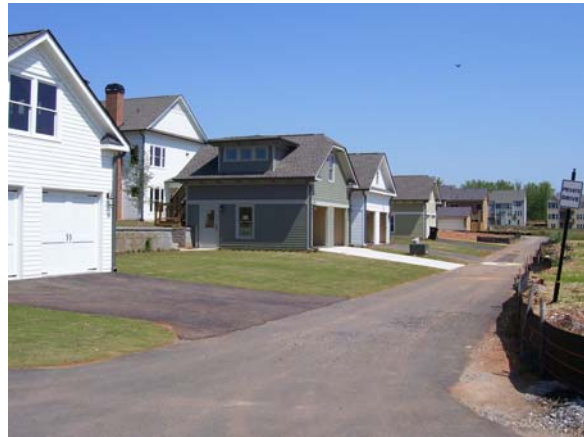
Rear (Alley) View Single-family Dwellings in South Village Harmony on the Lakes
