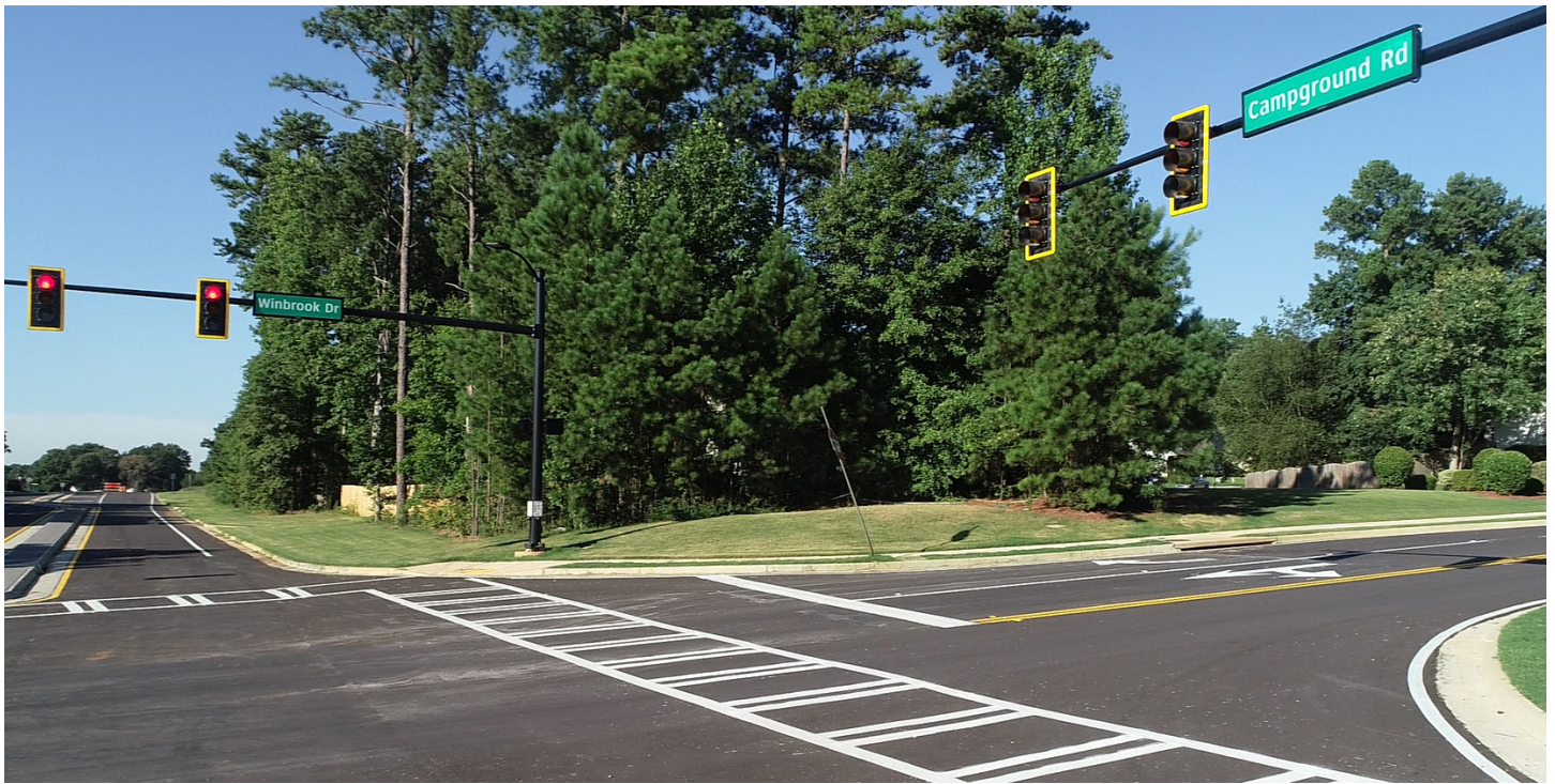
Intersection improvement at Campground Road and Winbrook Drive
