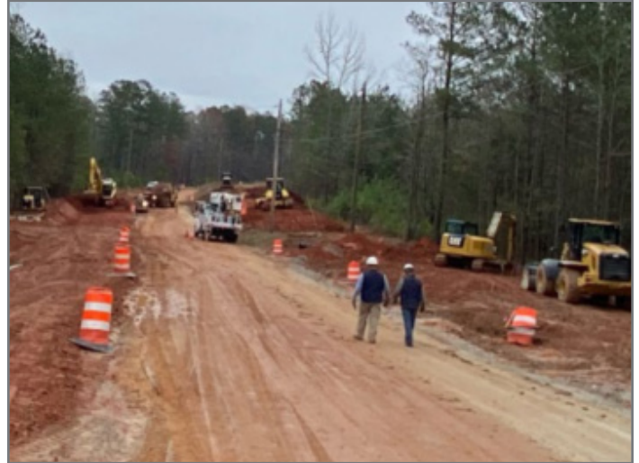
SPLOST roadway project under construction
