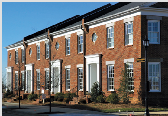
Form-based design guidelines promote a preferred development pattern by focusing on basic building dimensions and site layout rather than decorative features and materials that can increase costs.
