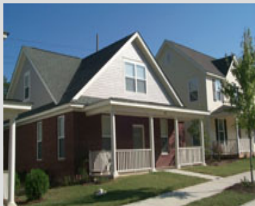
Form-based design guidelines promote a preferred development pattern by focusing on basic building dimensions and site layout rather than decorative features and materials that can increase costs.
