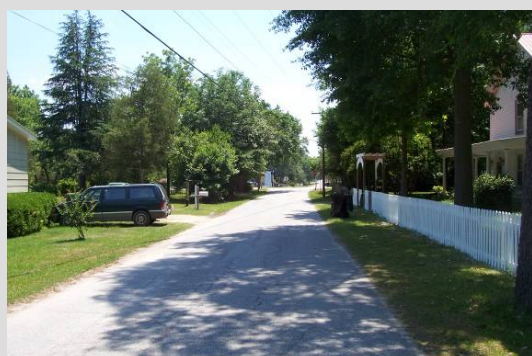
Lacking drainage channels and ponds that incorporate native vegetation to assist in storm water filtration; many existing Harlem neighborhoods experience problems with flooding along flat sections of street during heavy rain.
