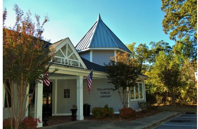
Figure 41: Public Library on Bowden Street
