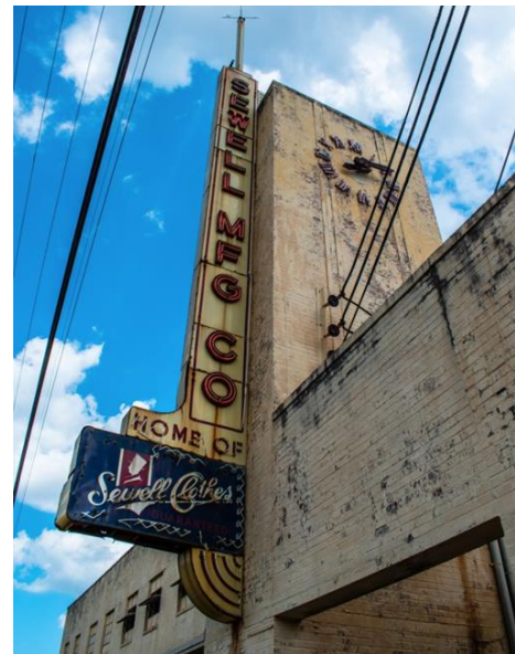
Figure 30: Historic Sewell Manufacturing Company building in Bremen
