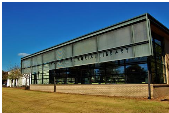
Figure 7: Warren P. Sewell Library in Bremen
