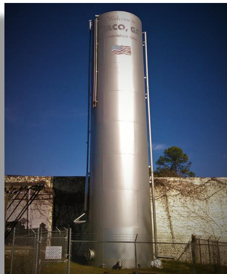
Figure 19: Water Tower in Downtown Waco
