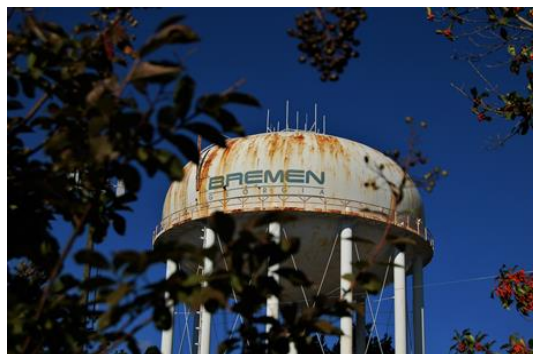
Figure 6: Water Tower in Bremen
