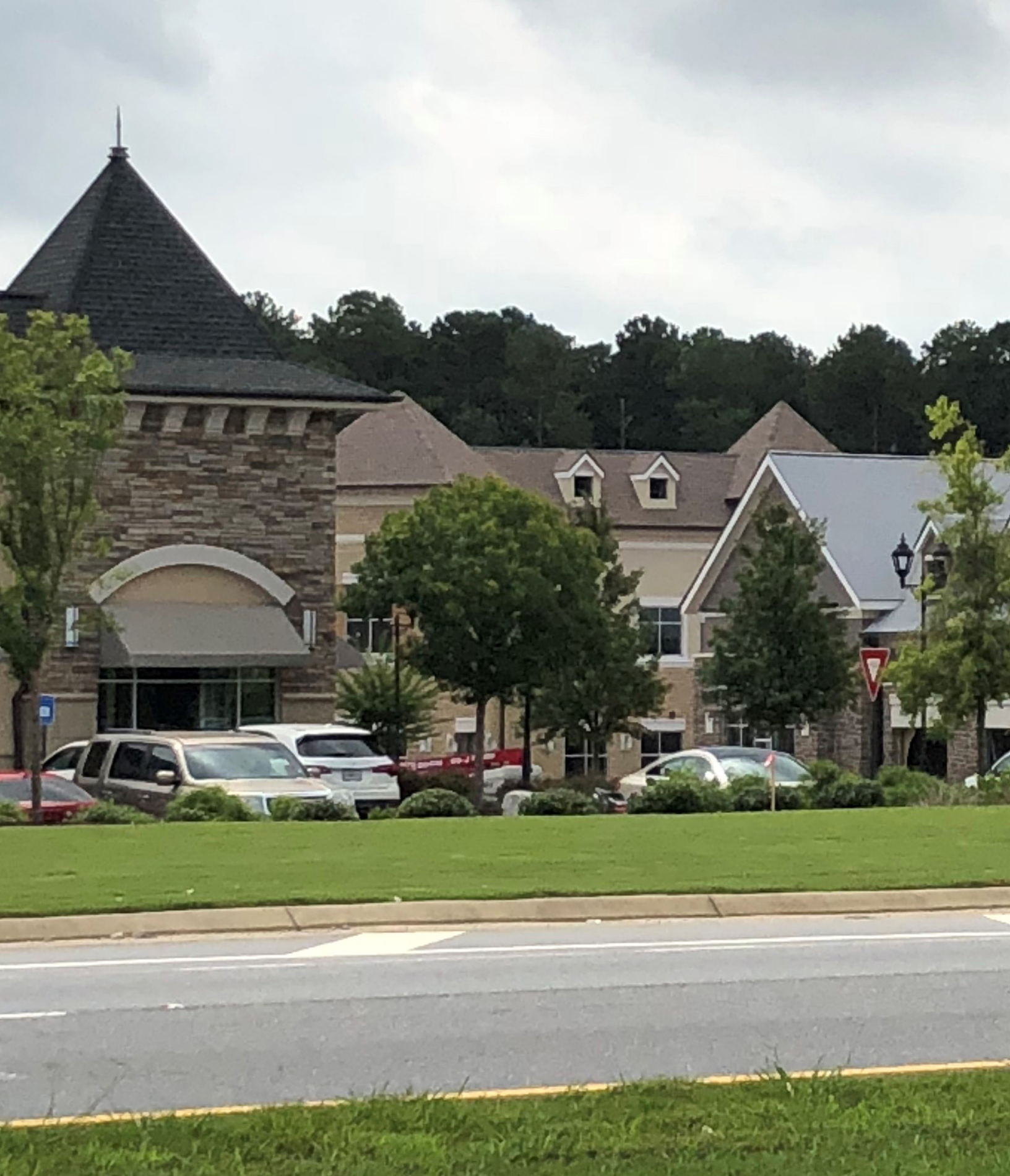
The in-progress Town Center development in Peachtree Corners
