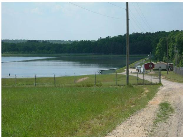
Grovetown’s sewage treatment facility is designed to take advantage of local soils to slowly filter waste water in a manner that reduces impacts on surface and ground waters.
