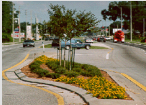
Landscaped medians and shared access can help improve highway efficiency but reducing the number of locations where vehicles can access travel lanes.
