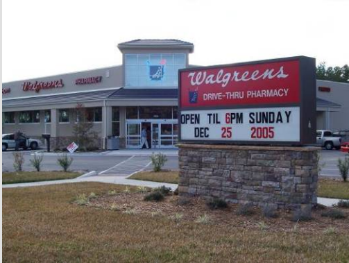
Reducing on-site impervious areas and the scale of commercial signage are just a few of many ways that Grovetown can guide community character.
