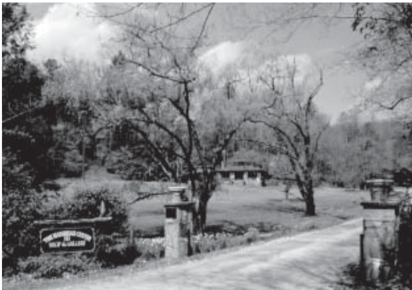
The Hambidge Center, located in the north Georgia mountains near Dillard, received two Georgia Heritage grants between 1997 and 2001, totalling $32,500 for rehabilitation work on both the Mary Hambidge house and the weave shed.
