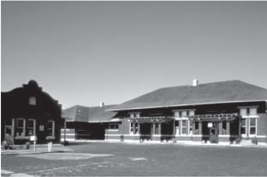
The Thronateeska Heritage Center in Albany houses its history museum in a 1912 railroad terminal, above.
