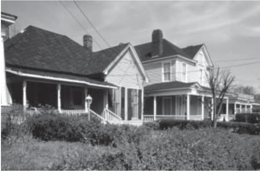
The Pleasant Hill Historic District is Macon's major historic African American neighborhood, featuring predominately one-story, simple, wood-framed houses that date from 1870–1930. The district was listed in the National Register of Historic Places in 1986.
