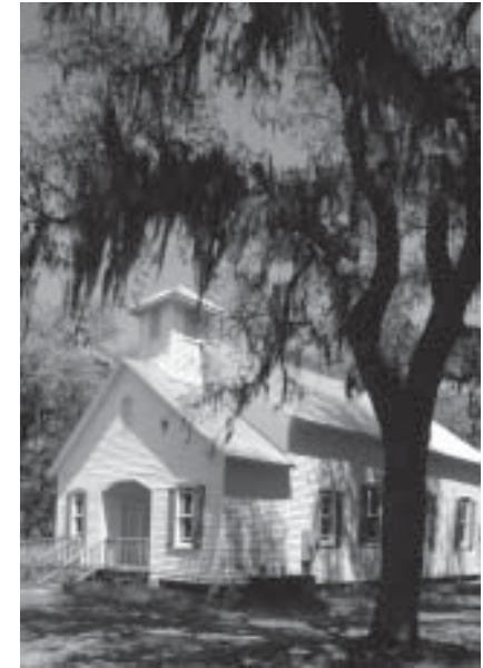
Raccoon Bluff Church, located on Sapelo Island, was built c. 1900. After being vacant for 40 years, the church was restored in 2000 with grants from the Georgia Heritage program and the Governor's Discretionary Fund.
