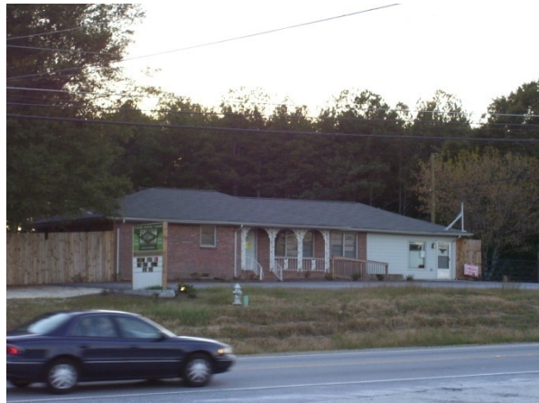
Commercial Use of Residential Structure Along SR 20
