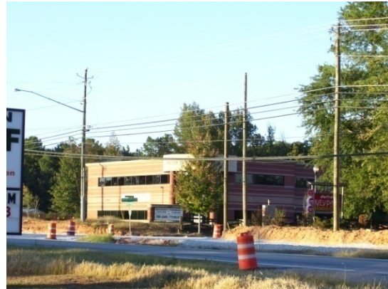
Office Building Under Construction, SR 20 Corridor, 2007
