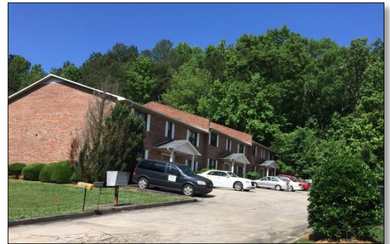
Multifamily housing, Calhoun.
