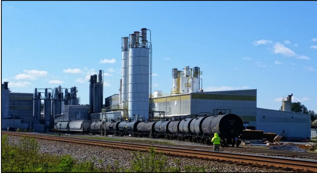
Huber Engineered Materials, Fairmount.
