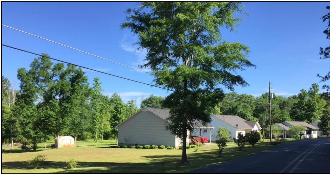
Franklin Road SW housing, Plainville.
