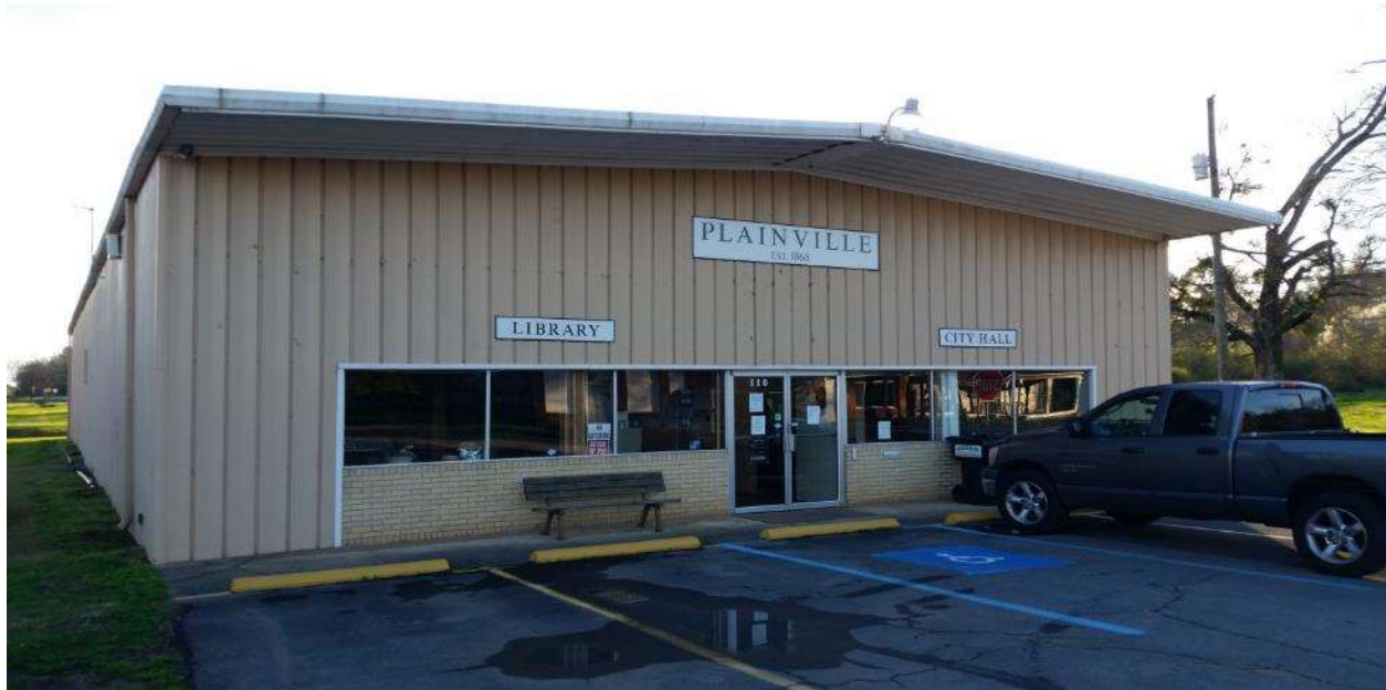
Plainville City Hall, Earl Street, Plainville.
