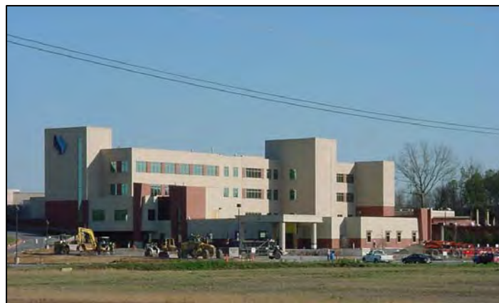
Gordon Hospital Expansion
