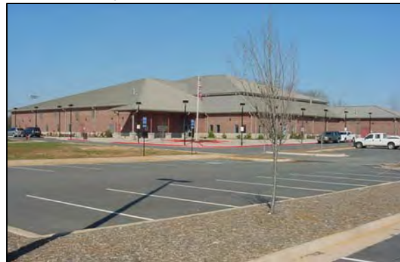
Sonoraville Recreation Complex
