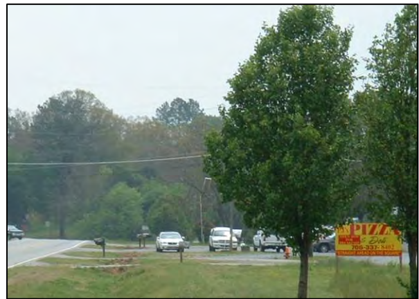
Separate driveways (versus shared) for commercial uses have the potential to impede traffic flow along U.S. Highway 411
