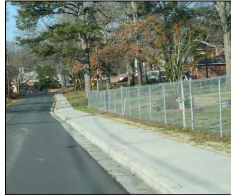
Sidewalks, like this one approaching Fairmount Elementary, provide important connections between neighbors, neighborhoods, and activity centers like parks and schools
