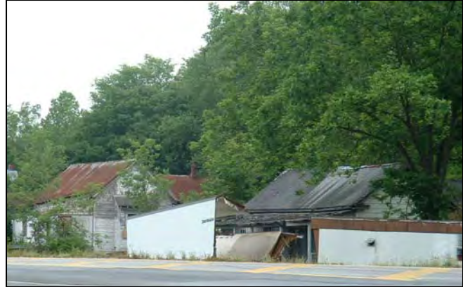
Disposal of junk and debris in the front yards of property along U.S. Highway 41 detracts from the character of the area
