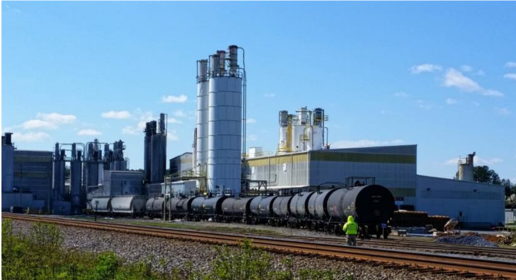
Huber Engineered Materials, Fairmount.
