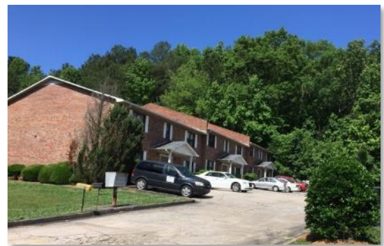
Multifamily housing, Calhoun.
