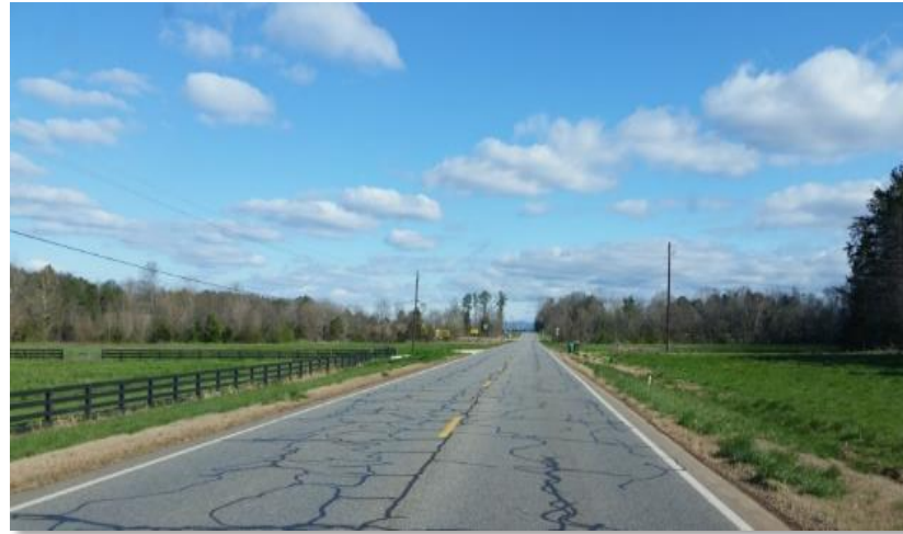
Highway 411 north of Fairmount.
