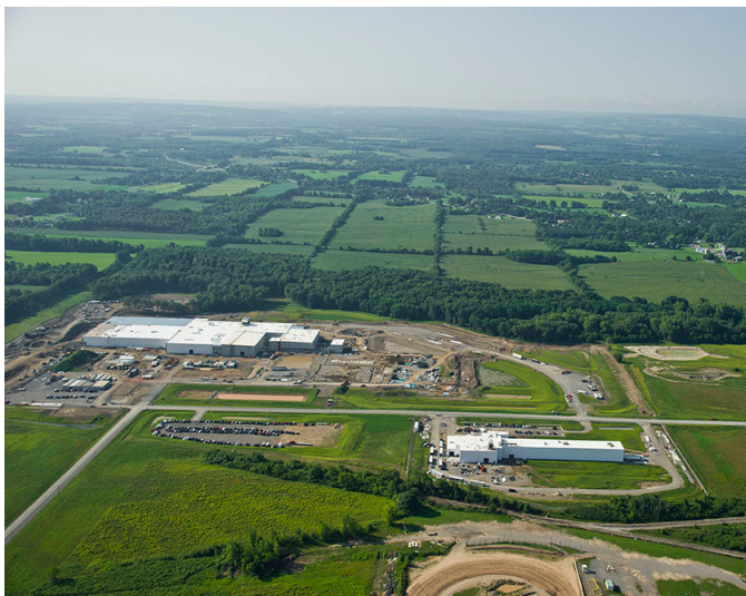
With adequate site planning and landscaping, industrial uses can fit in well into a rural landscape.
