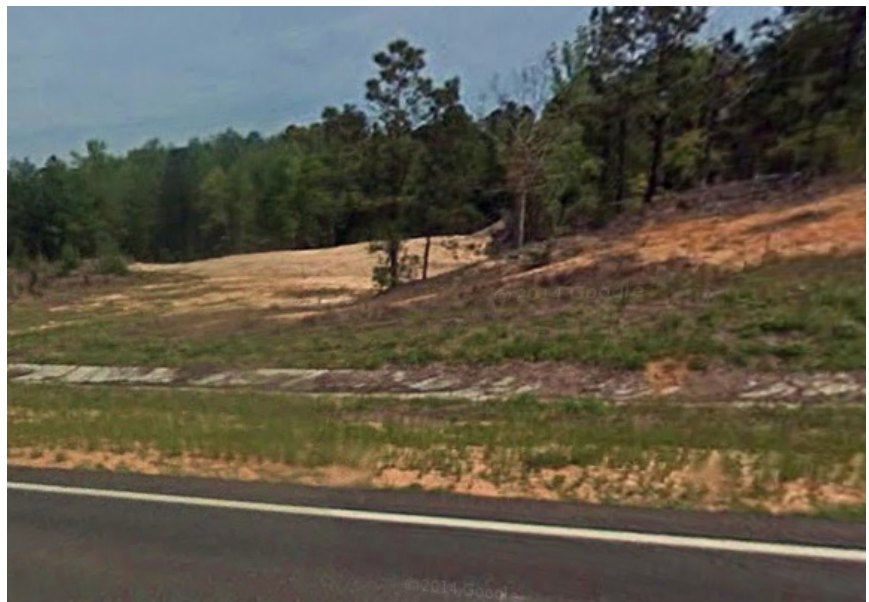
Glascocock County's industrial park property lies outside of Gibson on GA 102.
