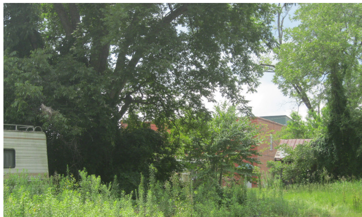
Building and property maintenance is an issue with some properties in this area.
