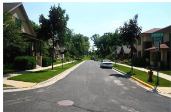
Curb and gutter along with pedestrian facilities and attractive landscaping provide this neighborhood with a unique sense of place
