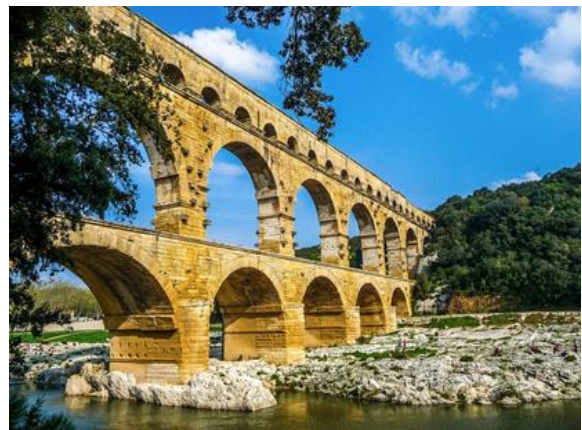
Figure 25: Historic Pont du Gard aqueducts in southern France illustrate that public drinking water infrastructure has been an important part of community design since the ancient Roman Empire.
