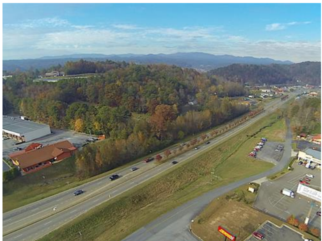
Figure 22: Aerial view of SR 515. Photo courtesy of the Ellijay-Gilmer Chamber of Commerce.
