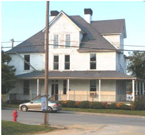
The Perry House, built in 1902 using timbers from the old Ellijay Hotel, will either be moved or demolished to allow for the construction of the new County Courthouse.
