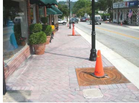
Sidewalks have been improved in Ellijay with Transportation Enhancement and local funding.
