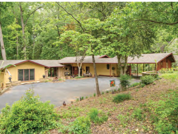
Located in Macon, Bibb County, the William and Jane Levitt House is an architect-designed ranch house with Contemporary styling of the Modern Movement that was retained in its recent rehabilitation.
