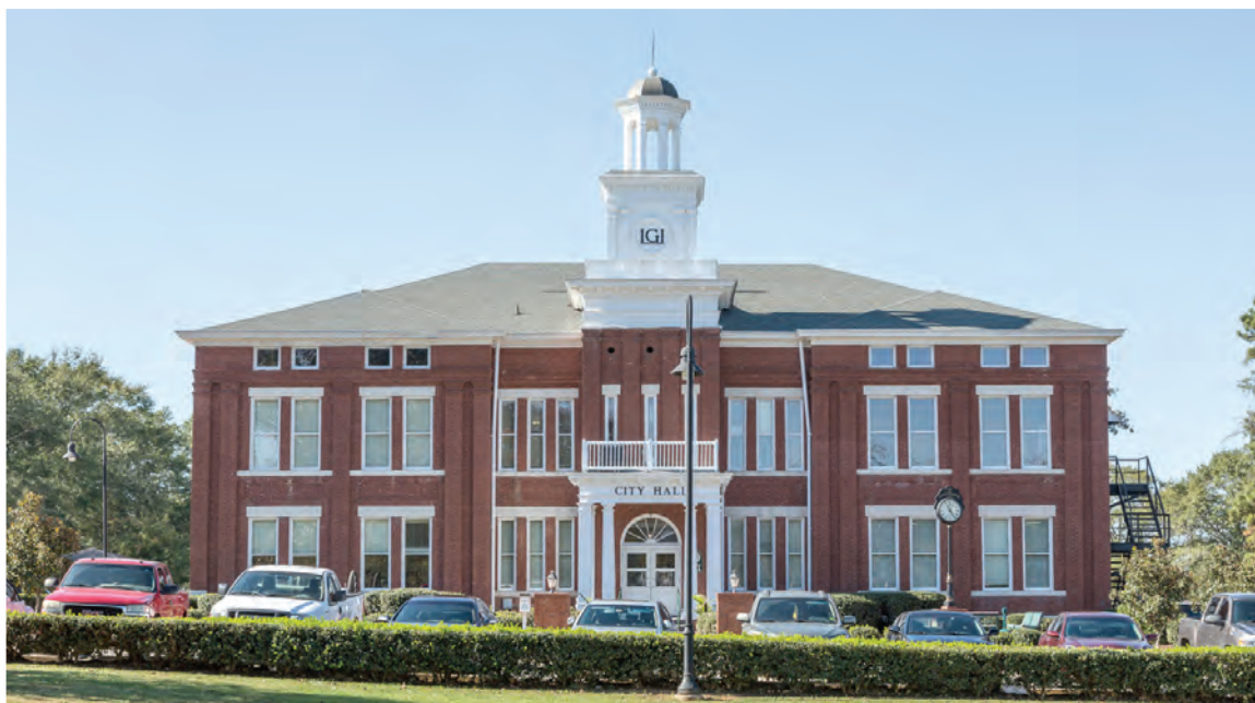
Originally a school, and now used as city hall in Locust Grove, Henry County, this is an excellent example of the preservation and adaptive use of a historic resource.
