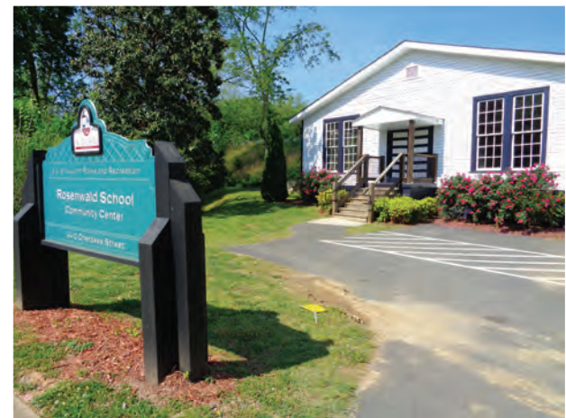
The rehabilitated Acworth Rosenwald School in Acworth, Cobb County. The school now serves as a community center.
