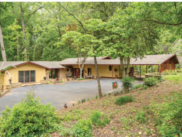
Located in Macon, Bibb County, the William and Jane Levitt House is an architect-designed ranch house with Contemporary styling of the Modern Movement that was retained in its recent rehabilitation.
