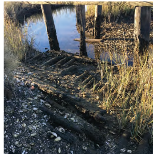
Roads are considered structures, as well as sites, as in this case of a historic Corduroy road located at Ossabaw Island.
