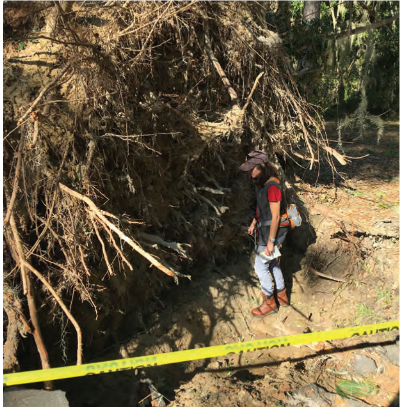
HPD staff assessed damage caused by Hurricane Irma at the Hofwyl-Broadfield State Historic Site in 2017.
