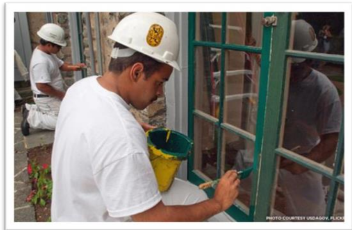
Workers Restoring Historic Windows
