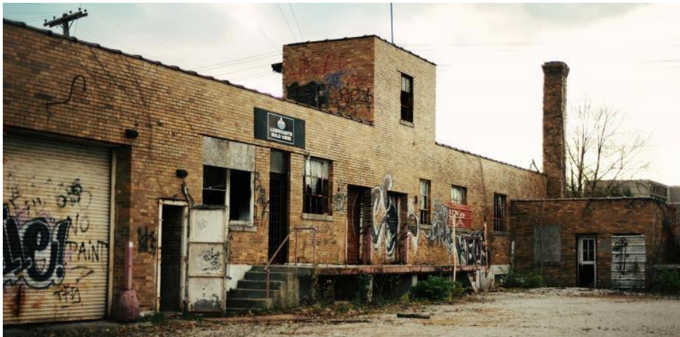
Example of a Brownfield
