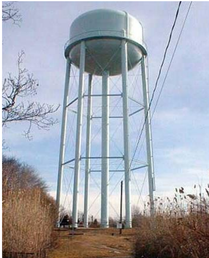
Example of a water tower
