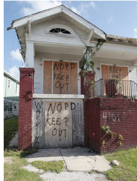
Neglected maintenance can lead to neighborhood blight
