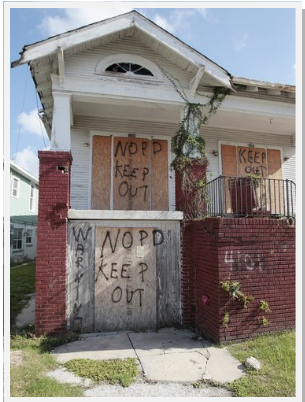
Neglected maintenance can lead to neighborhood blight
