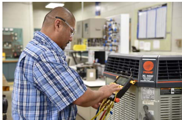
Technical College student learning HVAC repair
