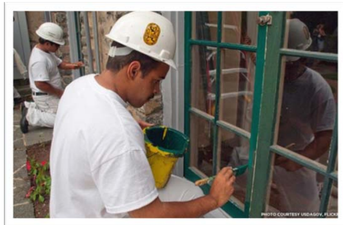
Workers Restoring Historic Windows
