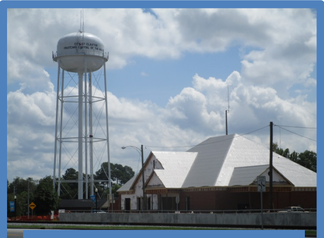
New City Hall under construction and water tank
