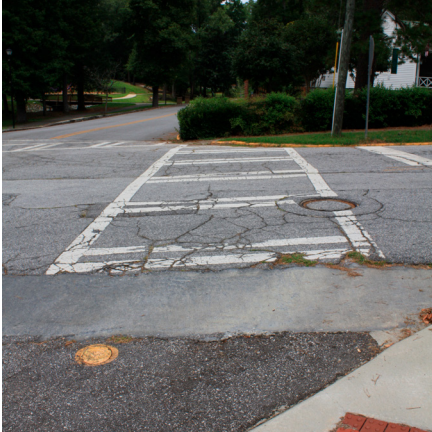
Image 9: Example of pedestrian crosswalk, Forest Avenue
