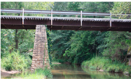
Image 11: Intersection of Mill Shoal Creek and King Hall Mill Road
