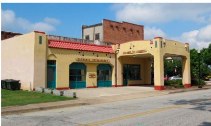
Image 6: Example of adaptive re-use for the Chamber of Commerce, Downtown Elberton
