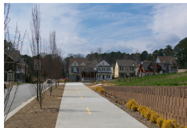
▲ New multi-use trail at Project Renaissance
