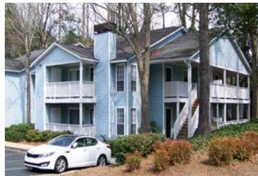
▲ Apartments off of North Peachtree Road
