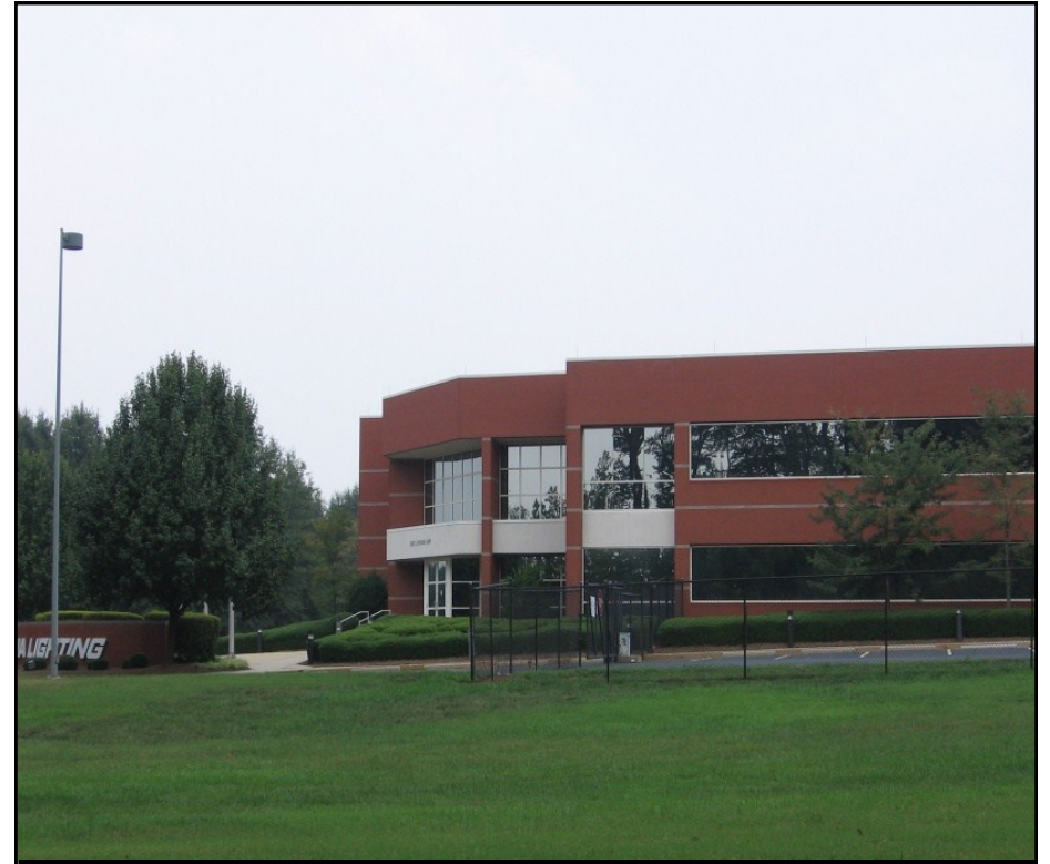
Typical office/distribution building.
