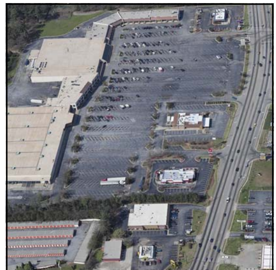
Large underutilized parking lot.
