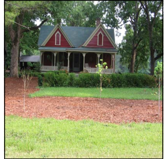
Rural home with traditional architecture in southeast DeKalb County
