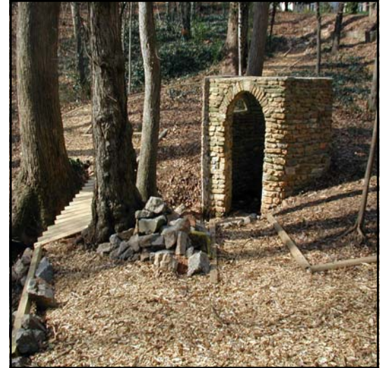
Historic Resource-Vernon Springs Well House.
