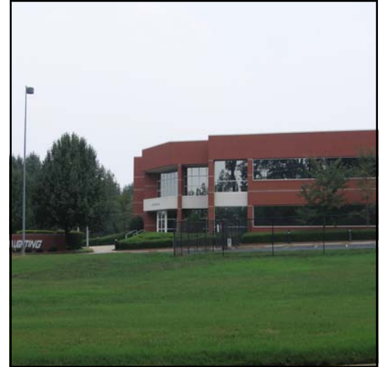
Typical office/distribution building.
