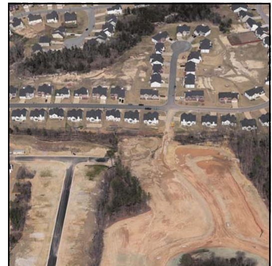
Suburban subdivision under construction with consistent lot pattern.
