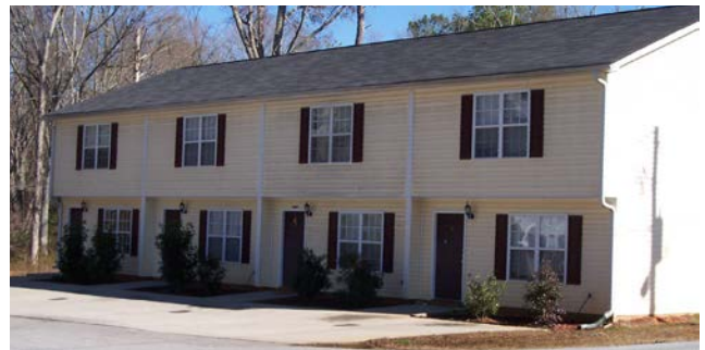
Figure 26 Source: Hall Consulting, Inc.
