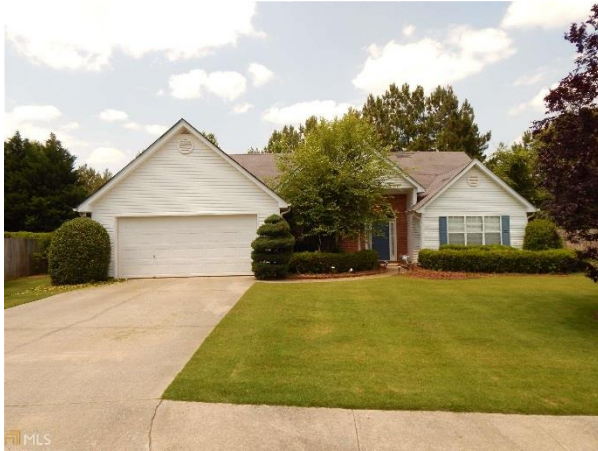
Housing on Nicholas Landing
