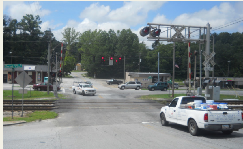
AT-GRADE RAILROAD CROSSING, DOWNTOWN DACULA
