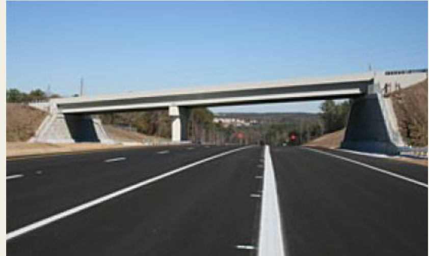
SUGARLOAF PARKWAY EXTENSION. PHOTOS BY AERIAL INNOVATIONS OF GA, LAWRENCEVILLE PATCH
