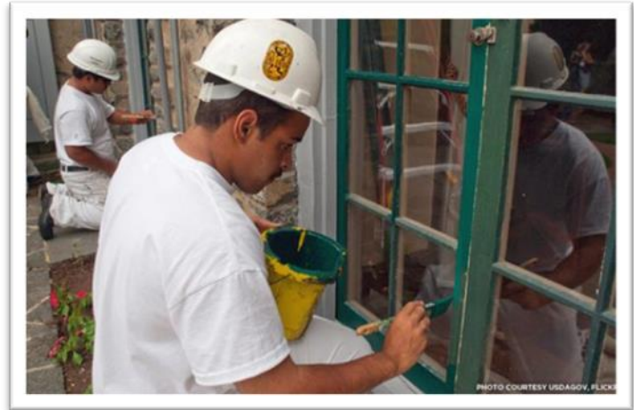
Workers Restoring Historic Windows
