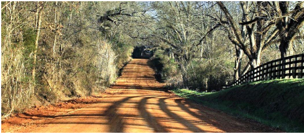
Dirt Road in Randolph County
