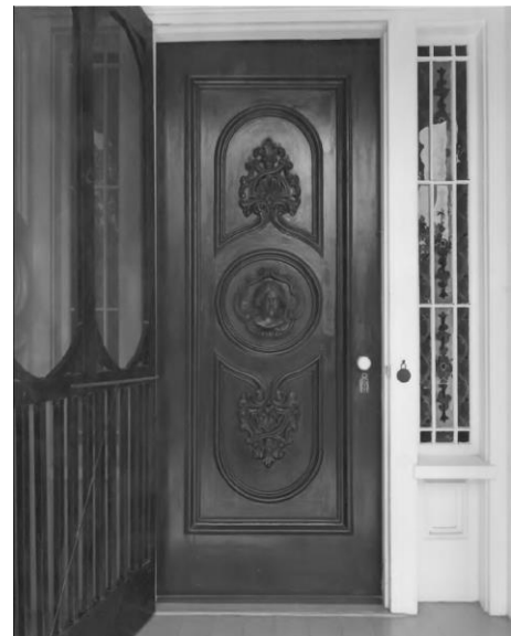
Sam Sawyer House Front Door Detail
