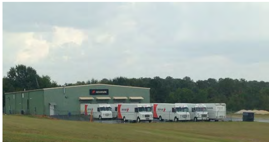
Figure 5: An example of a typical industrial use found in Crawford County.
