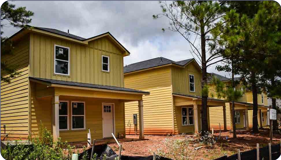
Image 28: Housing being built with CHIP funding by the Covington Housing Authority
