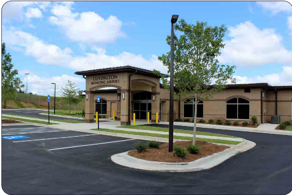
Image 20: Covington airport building
