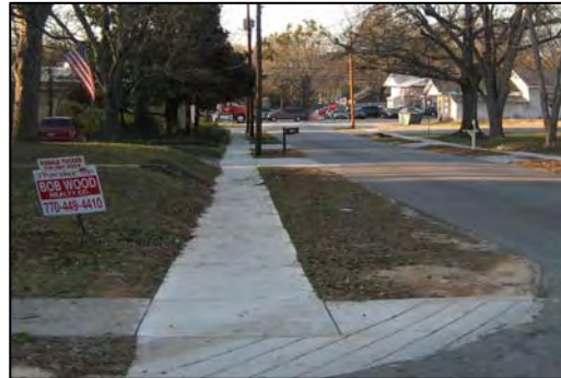
New sidewalks shown above provide improved pedestrian infrastructure in Winder
