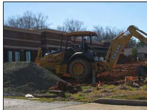
New strip commercial shopping centers under construction on Atlanta Highway in Auburn
