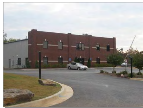
Existing industrial building in Statham
