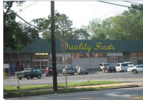
Strip mall located in north Winder near the SR 82/SR 53 split
