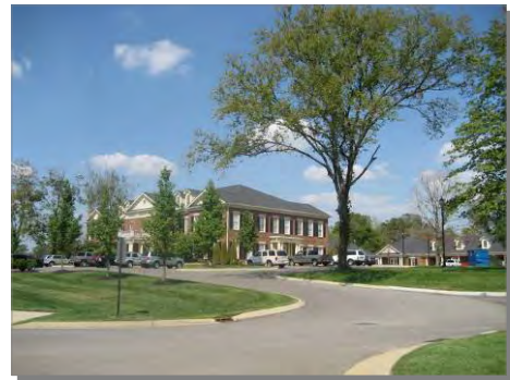
Redevelopment of Transition Corridors should preserve mature trees
