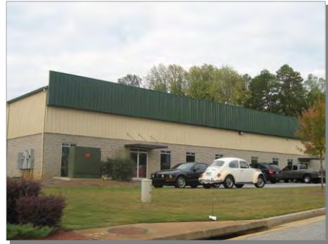
Existing industrial park building in Statham
