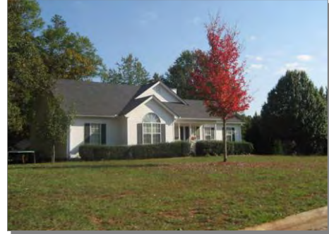
Single-family suburban home located in a west Bethlehem subdivision
