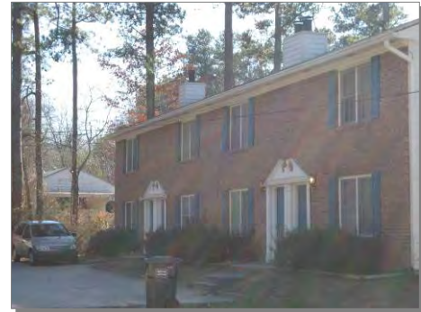
Multifamily housing provides housing choices near downtown Auburn
