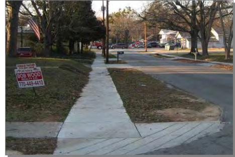
New sidewalks shown above provide improved pedestrian infrastructure in
