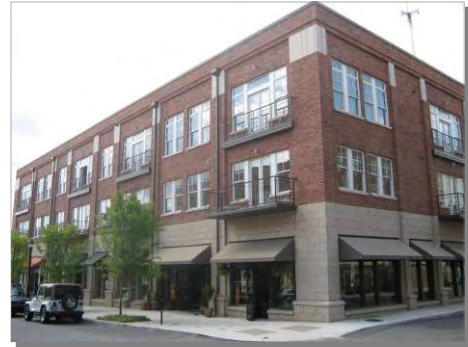
New construction in Downtown Winder should contribute to the existing historic commercial character
