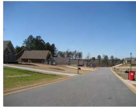
Suburban Neighborhoods in Barrow County developed for many years without sidewalks
