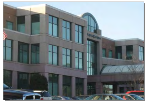
Barrow Community Hospital
