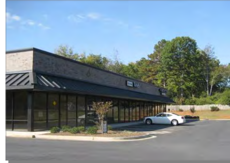
New commercial strip mall development located in Mixed-Use area south of Downtown on SR 11
