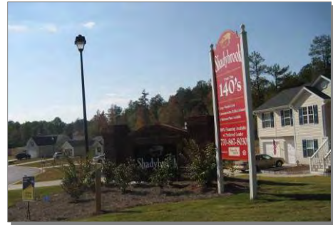
New home construction in unincorporated Barrow County
