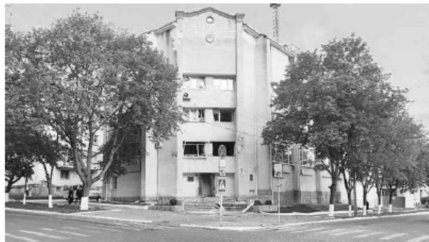
An explosion Monday damaged a building of the Ministry of State Security in Tiraspol, the capital of the breakaway region of Trans-Dniester, a disputed territory that borders western Ukraine. Police said several explosions in the territory were believed to be caused by rocket-propelled grenades.
