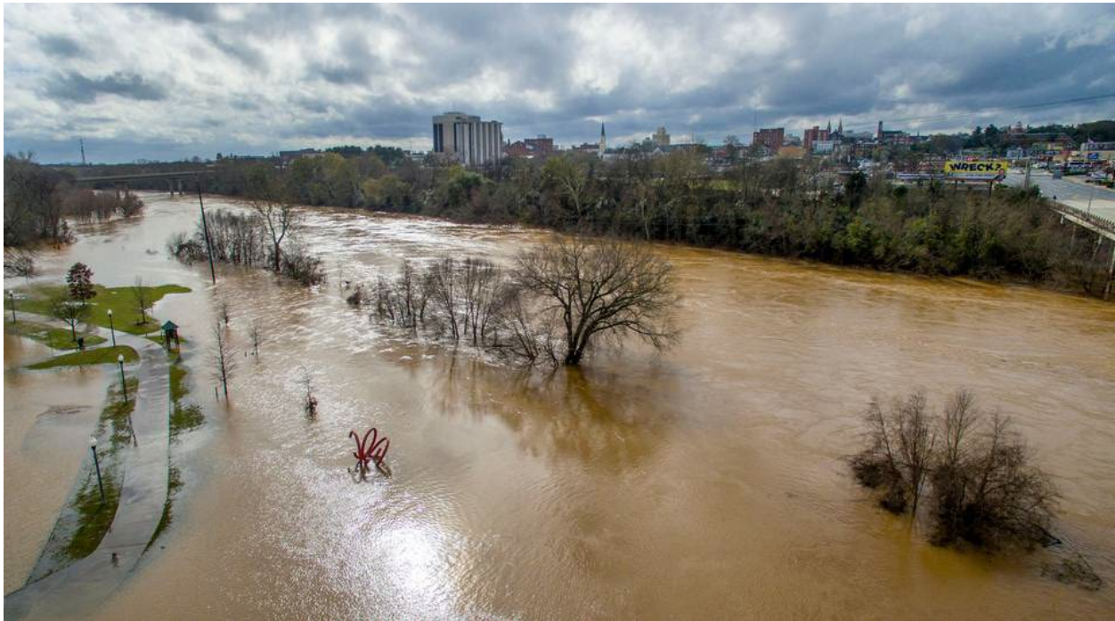
Figure 9-1: Ocmulgee River, Below Spring Street Bridge, at Flood Stage, December 28, 2015
